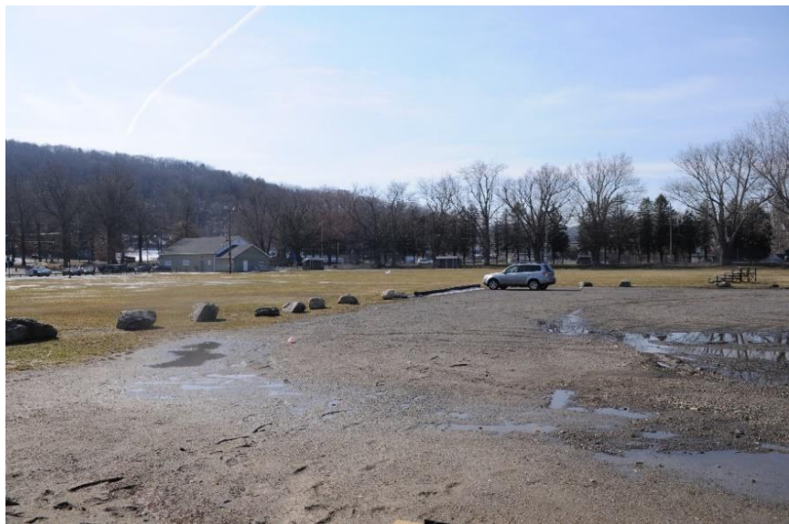
Figure 6. The dirt parking lot on the northern edge of Rowley Field becomes muddy when it rains and would benefit from proper drainage and/or permeable pavement.
